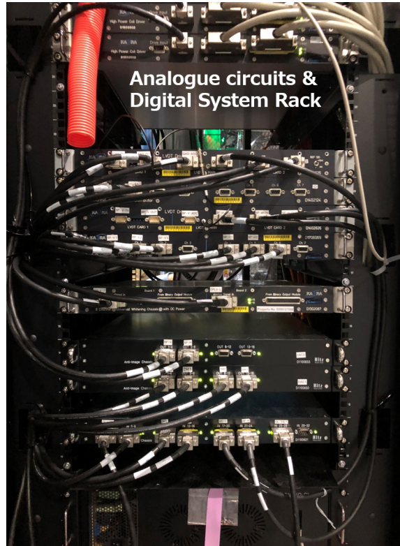
Figure 4.35: An example of in-air cabling.
