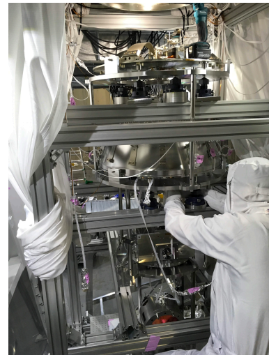
Figure 4.4: Installation of the Standard Filter.
