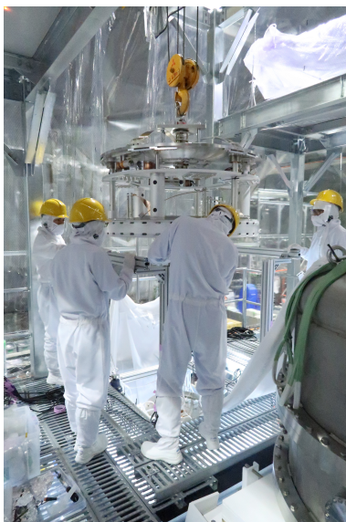
Figure 4.5: Installation of the Preisolator.
