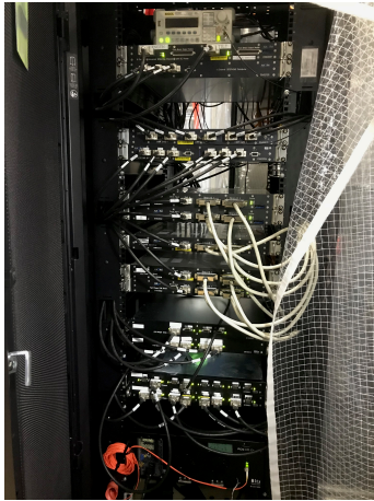
Figure 4.7: This is a rack for analog circuit and digital system.
