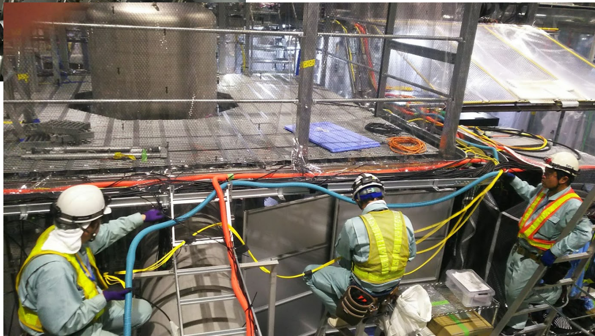
2018 summer; Installation of optical fibers by Fujitsu FSAS
