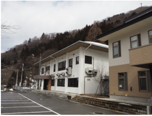
Hokubu-kaikan (Left building) was renovated for KAGRA.
