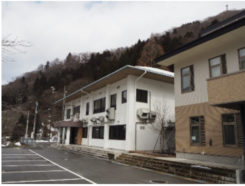
Hokubu-kaikan (Left building) was renovated for KAGRA.
