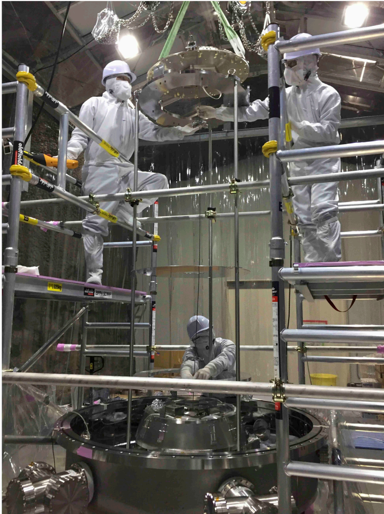
Installation of type-A on 2 nd store at Y-end
