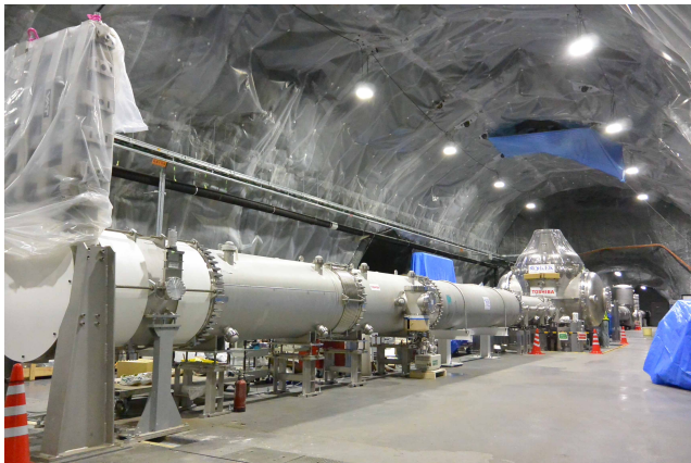
Completed X&Y front
