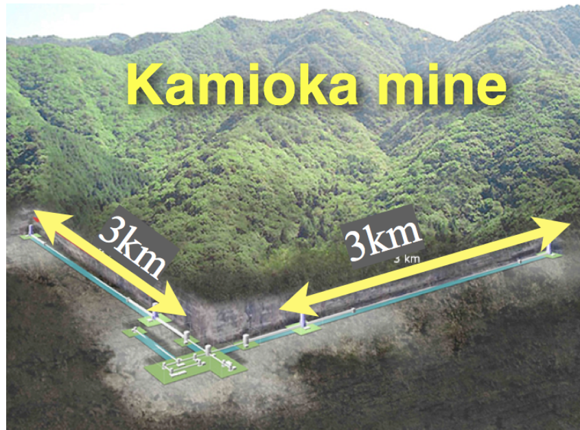
Figure 2.5: Image view of KAGRA in the Kamioka mine. KAGRA which has 3 km length arms is under construction in the Kamioka mine.
