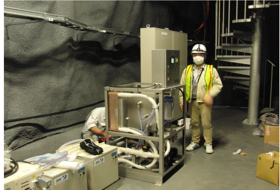
Piping for cooling water
