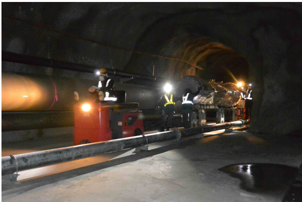
Duct shield transportation
