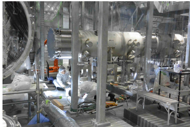
Duct shield installation
