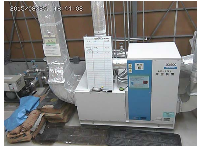
Fun hut (tunnel entrance house)
