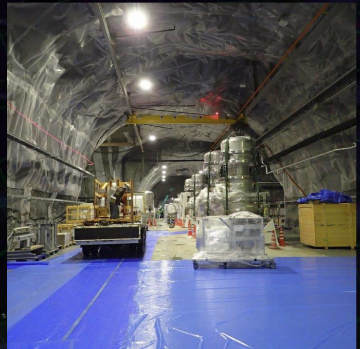
Center Cavern (March 2015)
