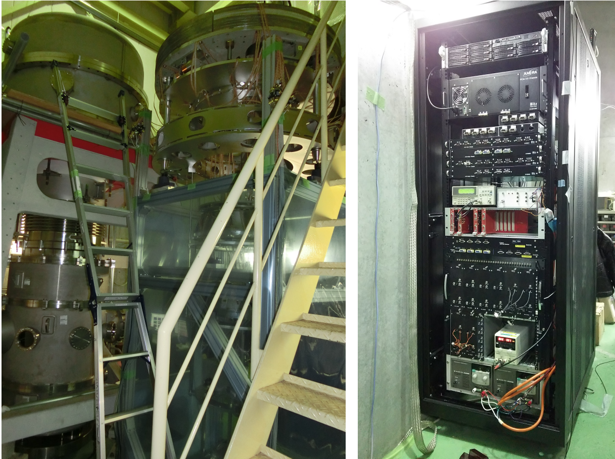
Figure 7.2: ( Left ) The type-B SAS prototype on an assembly frame waiting for installation into the vacuum chamber on the left. ( Right ) A rack containing digital system and analogue circuits for sensors and actuators. Electrical cables from the suspension system have not been connected yet.
