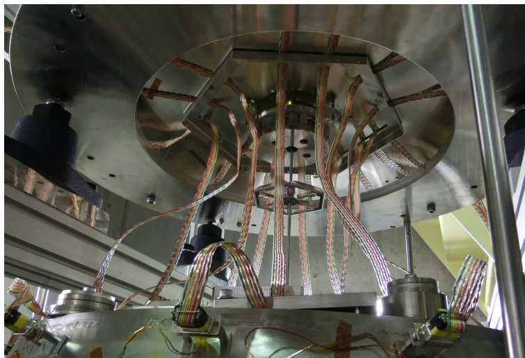
Figure 7.15: A picture displaying electrical cables between BF and F1. Rainbow-colored ribbon cables are clamped to the suspension stages and arranged loosely between them.
