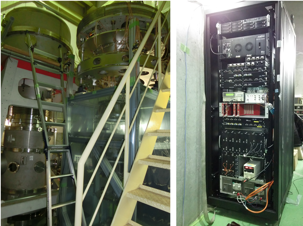
Figure 7.2: ( Left ) The type-B SAS prototype on an assembly frame waiting for installation into the vacuum chamber seen on the left hand side. ( Right ) A rack containing digital system and analogue circuits for sensors and actuators.
