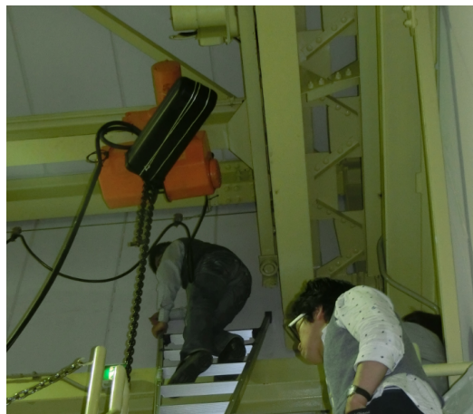
Fig. 5: A chain-holder (black cuboid) brought up by a plastic rope
