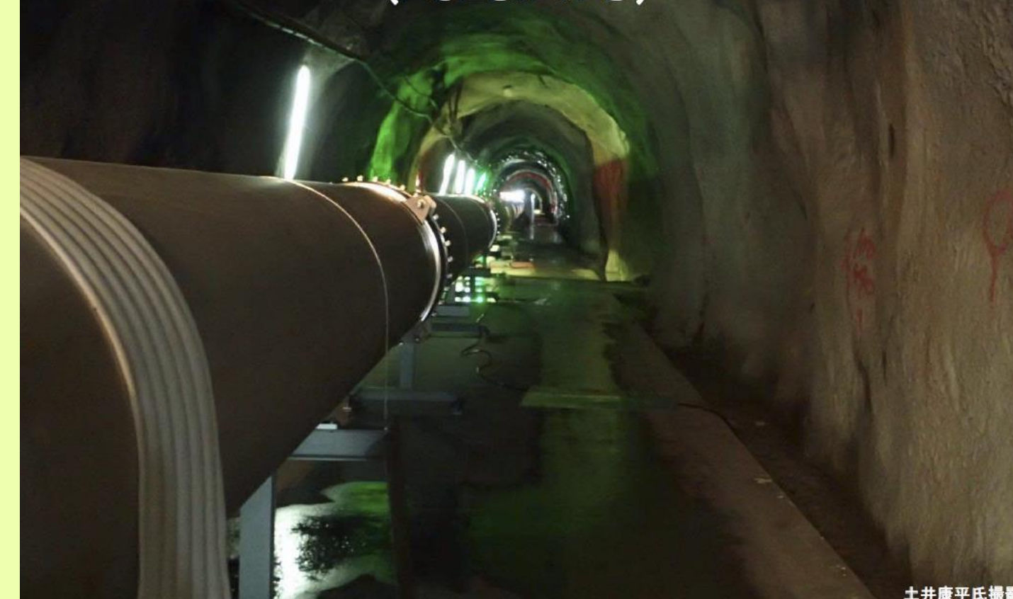
underground tunnel and 3-km vacuum pipe (2015.2.13)
