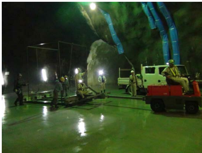
Assembling a mock-up gauge on a low-floor cart
