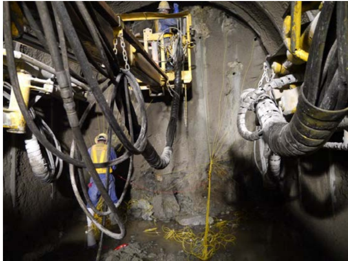
Preparation of blasting
