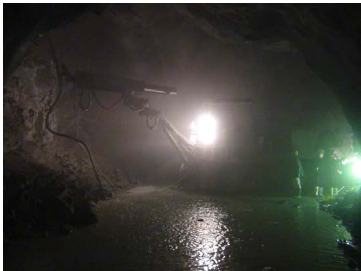
Shotcrete (spray gunite)
