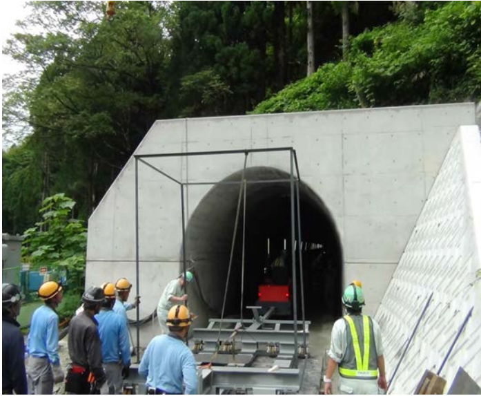
Assembling a mock-up gauge on a low-floor cart
