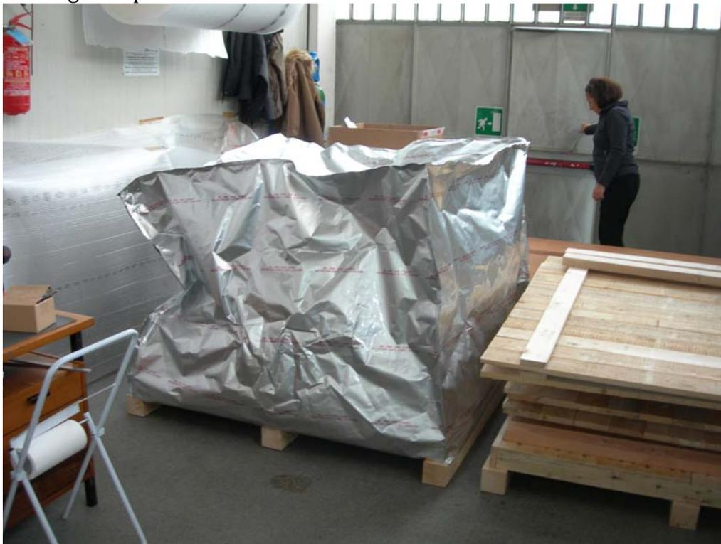
At the end the side panels of the shipping crate are screwed on the sides of the base, then two spreader beams, and finally the cover of the crate is screwed in place. Two pre-isolator filters per box are ready for shipment. Three crates for a total of six pre-isolator filters will be shipped in 2013.
