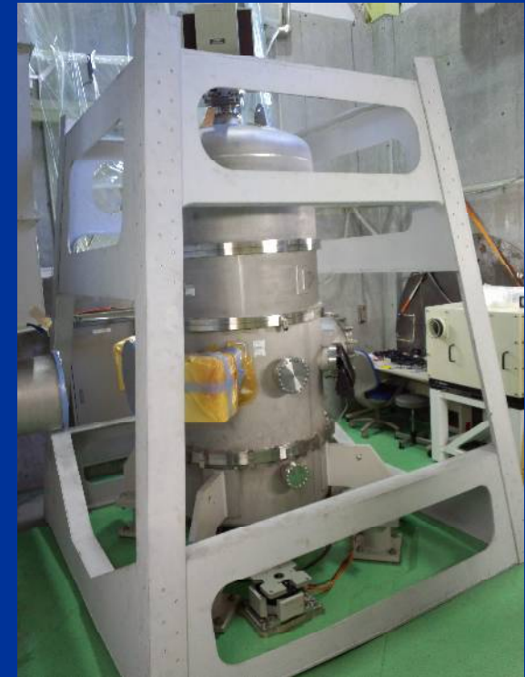
Outer frame installed in February, 2013.
