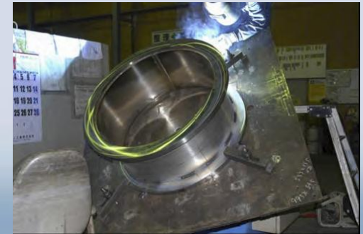
Welding on the connection port
