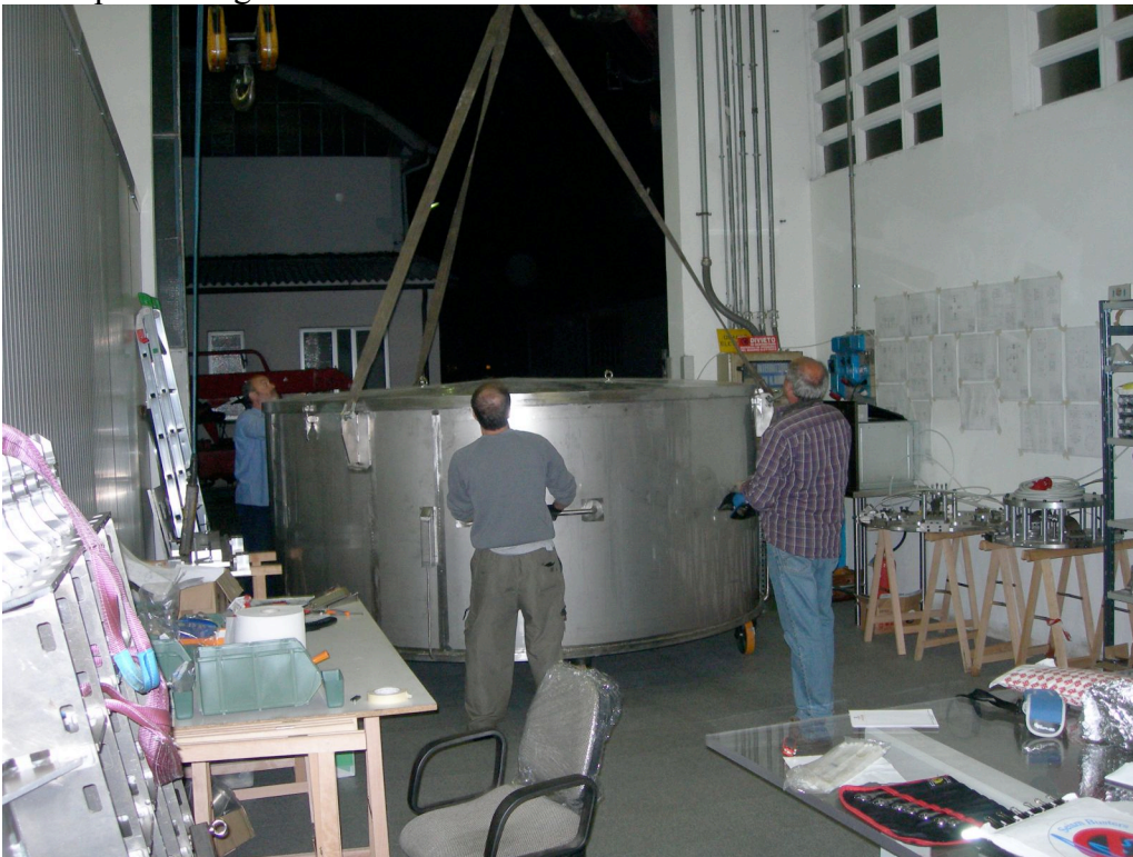
The large (3 m diameter) clean Bake-out oven entering the grey room.
