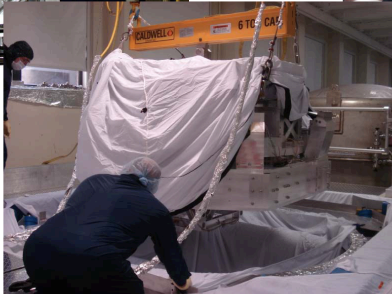
April 2008 – Quad-ISI BSC installation
